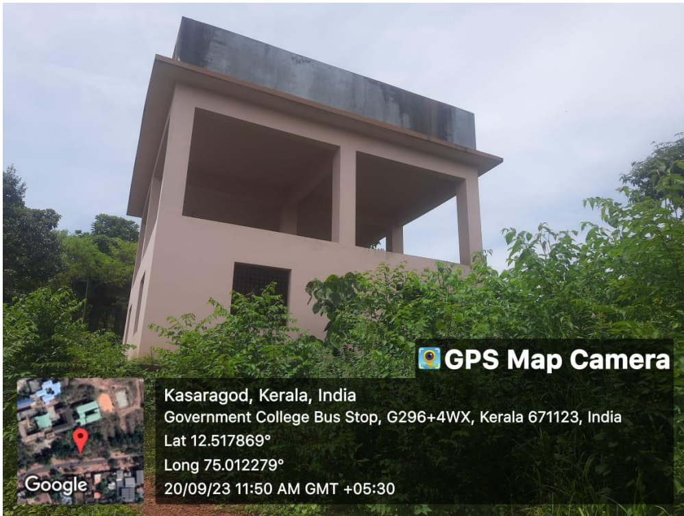
water storage tank
